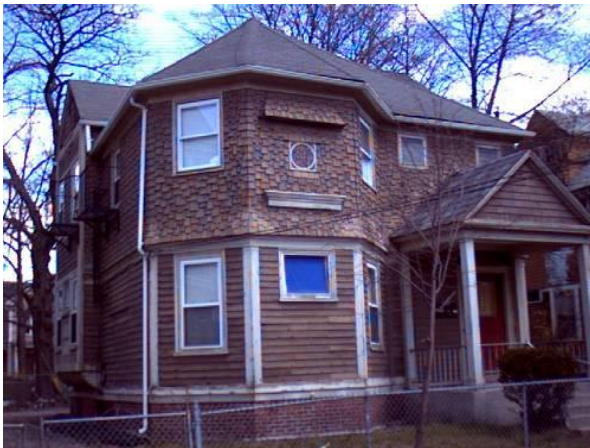
Typical foreclosure at 117 Daboll Street
