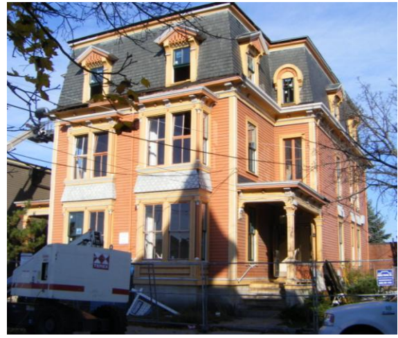
53 Parkis under renovation
