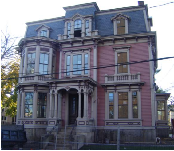
14 Parkis under renovation
